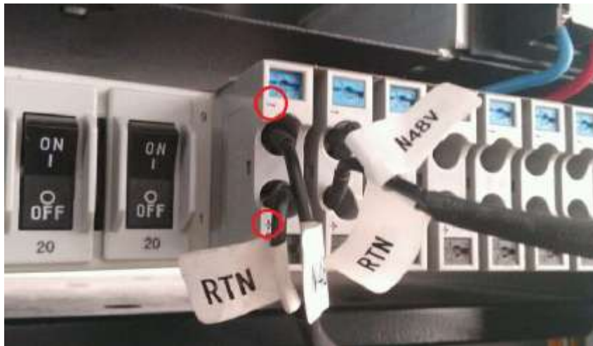
Figure 0-3 DC Power Cord Connection Diagram
